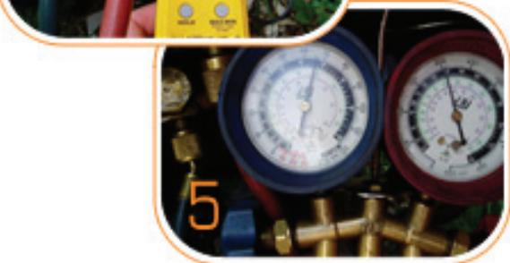
6: Set Suction Line Pressure. Read Required Suction Line Temperature opposite Required Superheat.
